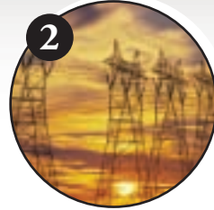
2 Large transmission lines move electricity from power plants at high voltage.
