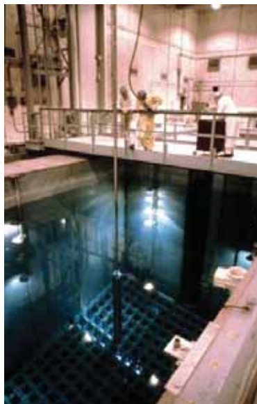
Spent Fuel Pool
