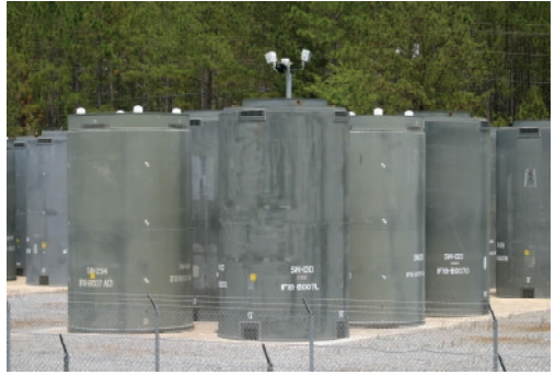
Dry storage at Plant Hatch.
